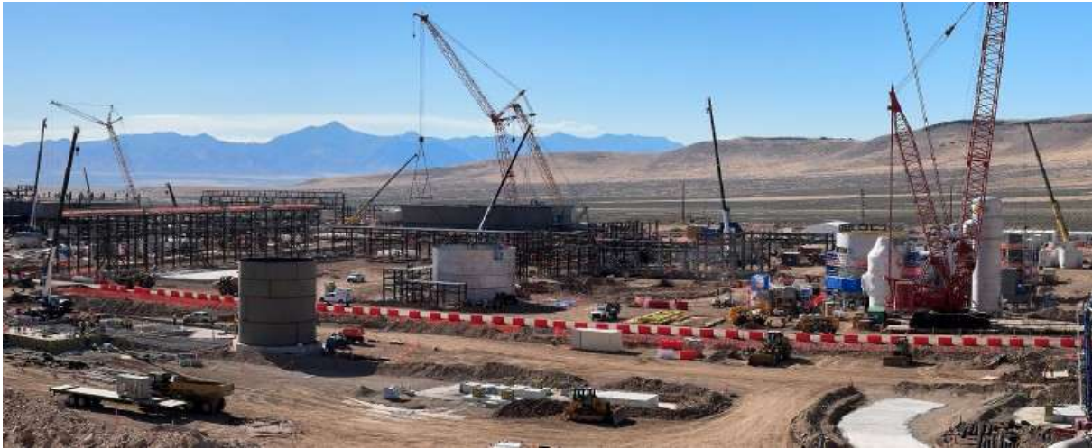
Construction progress at Thacker Pass
