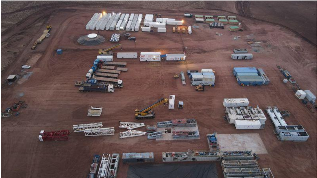
Figure 2 - Musuma-1 wellsite and rig camp aerial view
