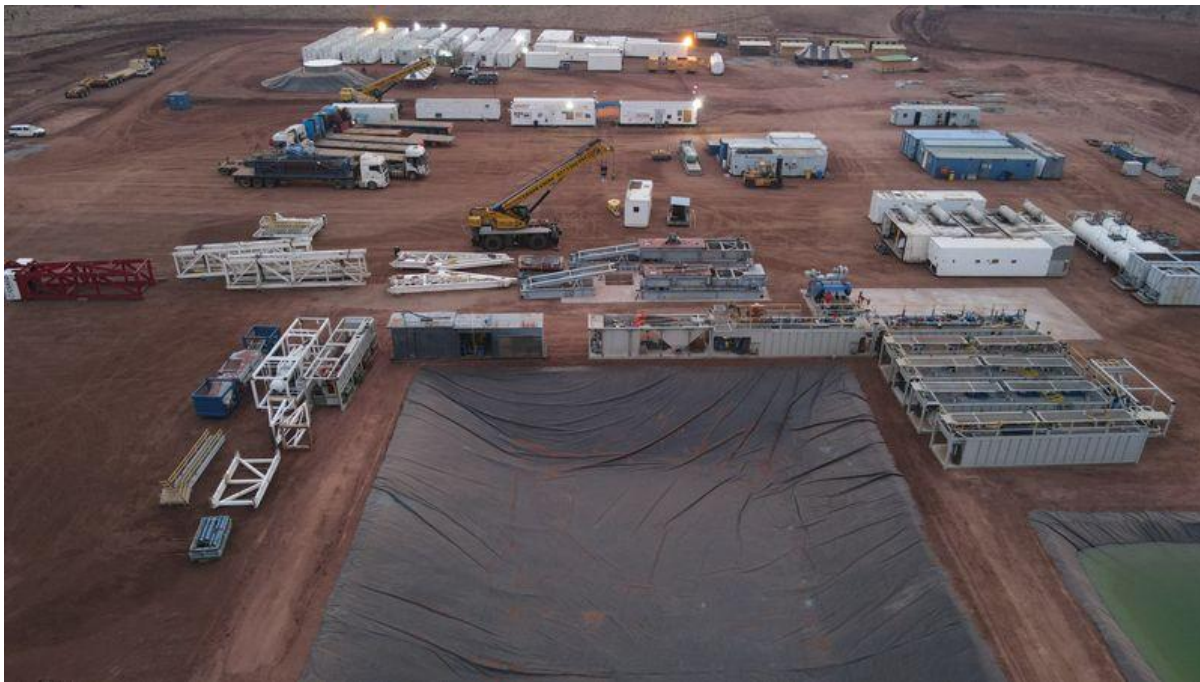
Figure 1 - Musuma-1 wellsite with Rig 202 substructure and mast preparation for rig-up
