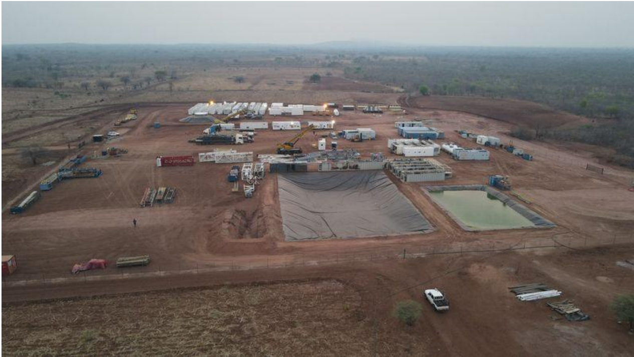
Figure 4 - Musuma-1 wellsite aerial view
