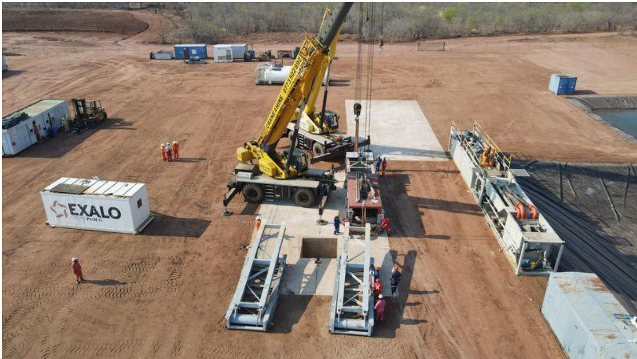
Figure 3 – Rig 202 substructure installation preparation
