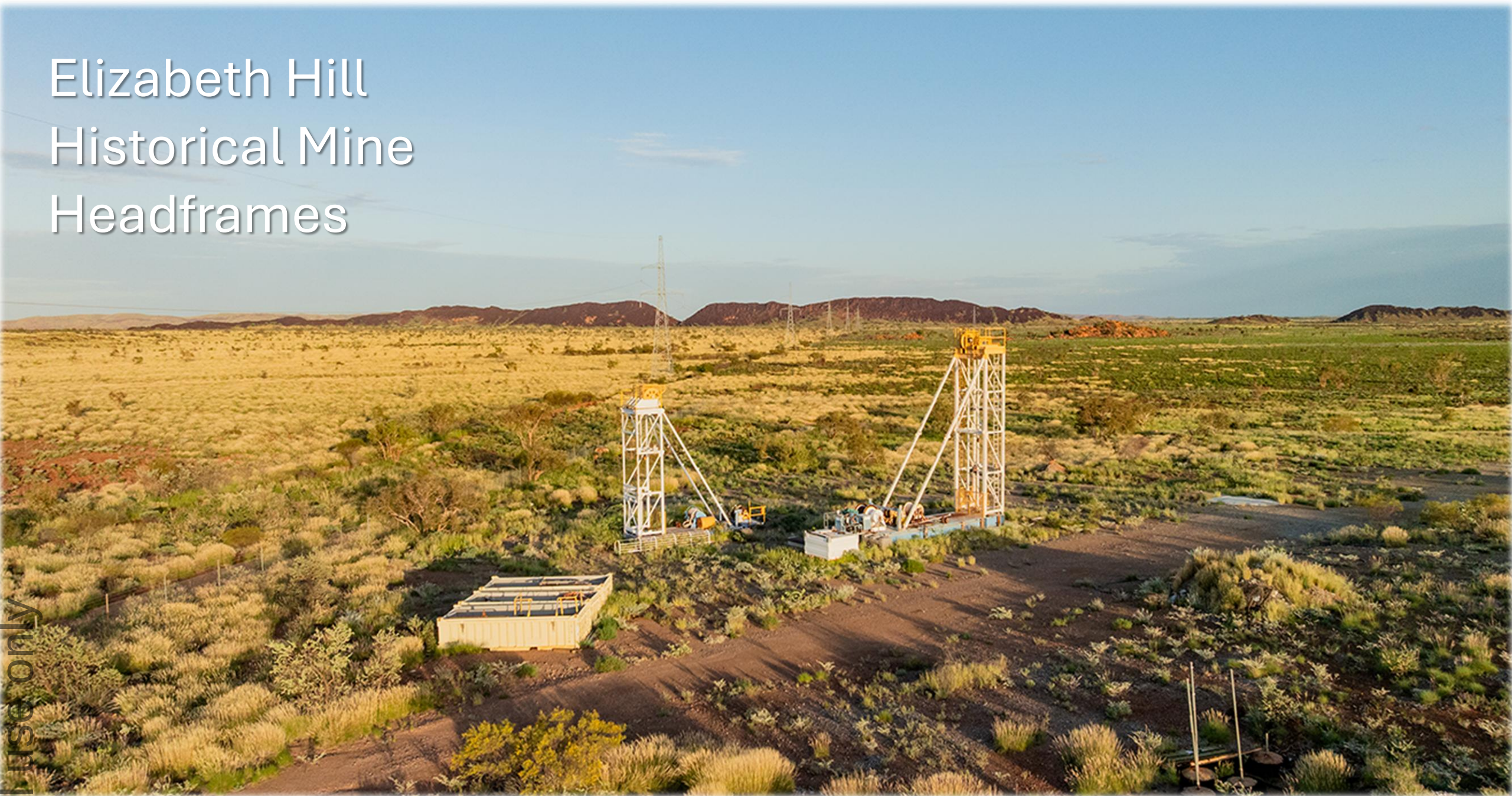
Elizabeth Hill Head Frames: Historic mine infrastructure at the high-grade Elizabeth Hill Silver Project, where drilling is targeting extensions to the known silver mineralisation along the Munni Munni Fault.
