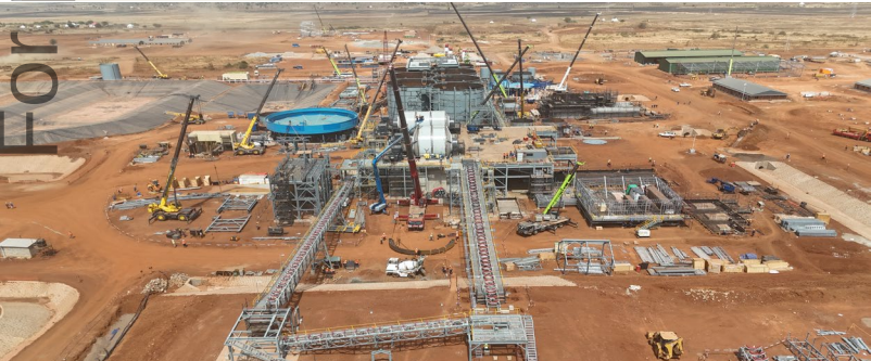
Process plant construction
