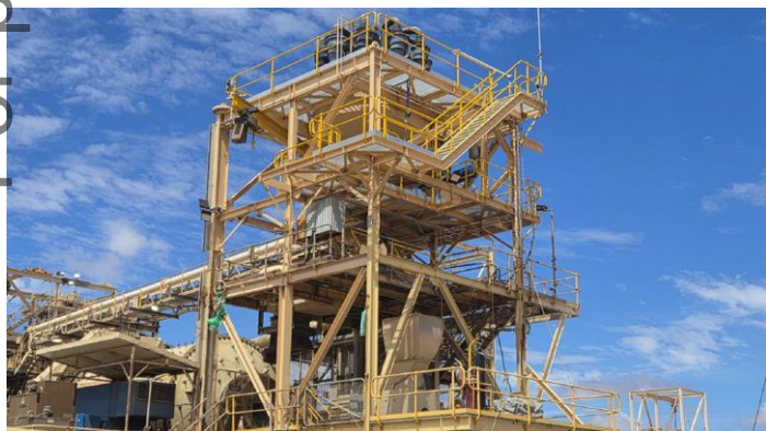
Figure 12: New cyclone tower structure in place
