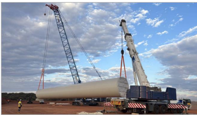
Figure 13: Wind turbine tower section lift
