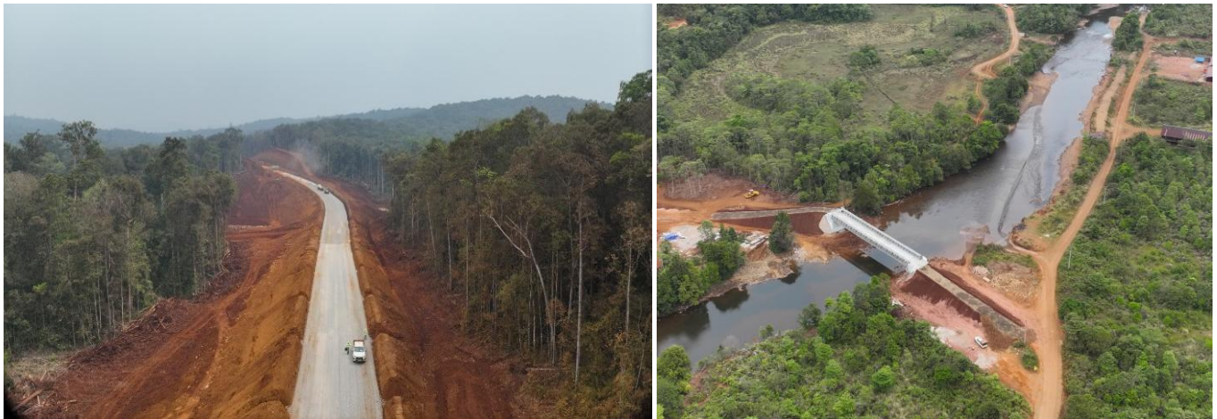
Sampala Mine construction activities
