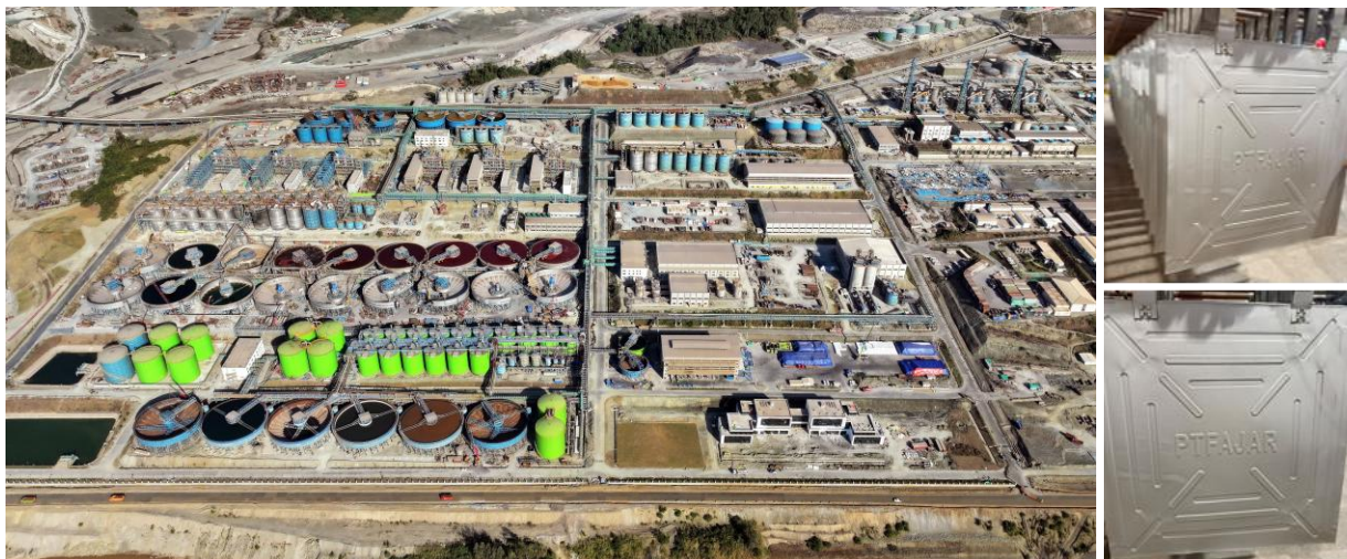
ENC, TMI and CNE HPAL Smelter complex and Fajar branded cathode
