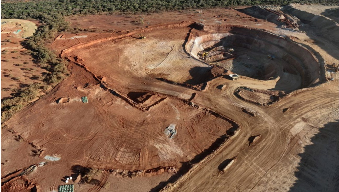
Figure 3: Cloudkicker open pit at the end of September 2026
