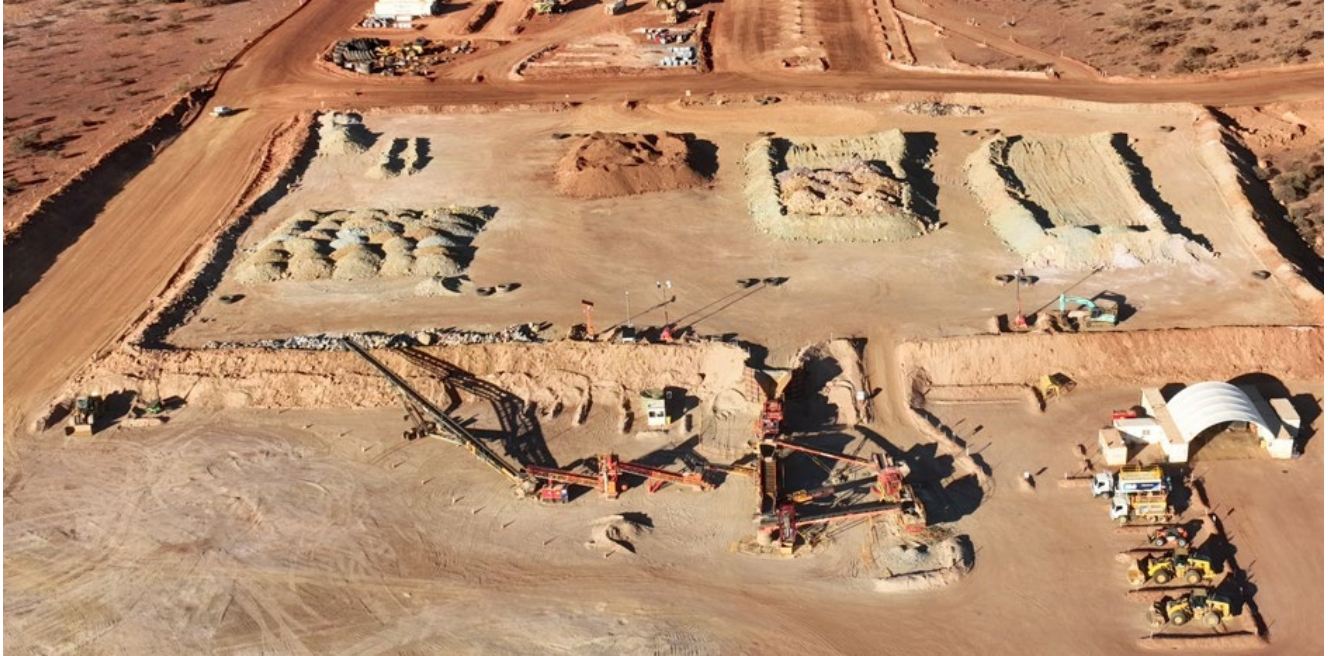
Figure 4: Crown Prince Gold Mine ROM, Crusher and Crushed Ore product stockpile area
