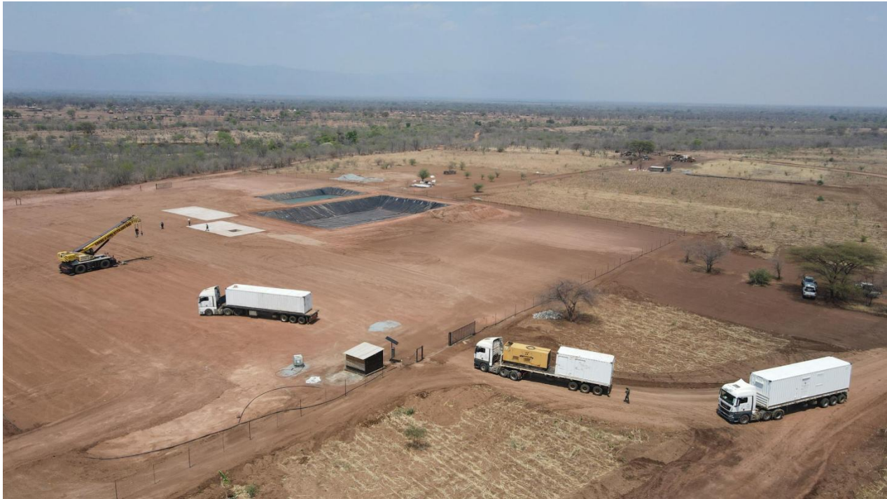
Figure 3 – Arrival of first load of Rig 202 camp
