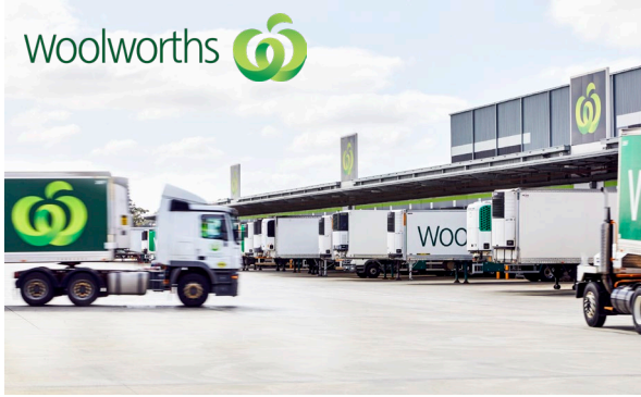
Woolworths Distribution Centre, Melbourne
