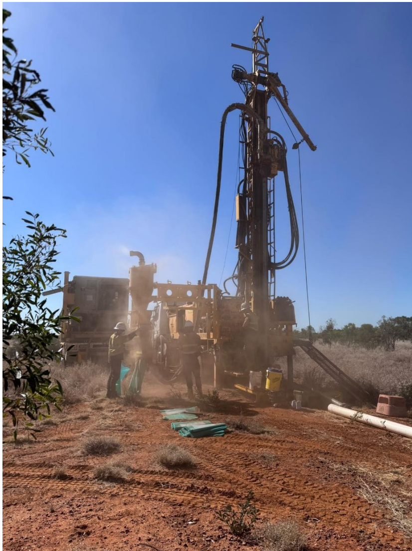
Figure 1 – RC drilling underway at the Rochedale rare earth prospect, Sybella-Barkly Project, northwest Queensland.
