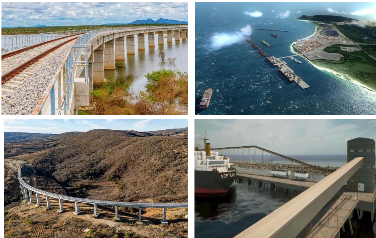
Figure 3: Fiol Rail (70% Complete), Porto Sul (Design)
