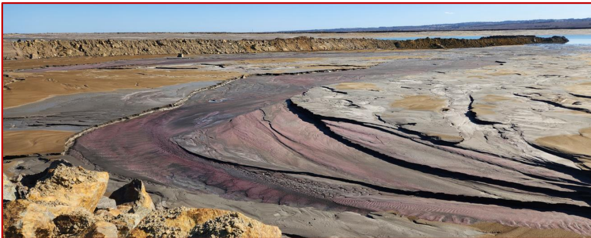
Figure 4: Kanmantoo tailings storage facility - the garnet-bearing tailings the Company will retreat
