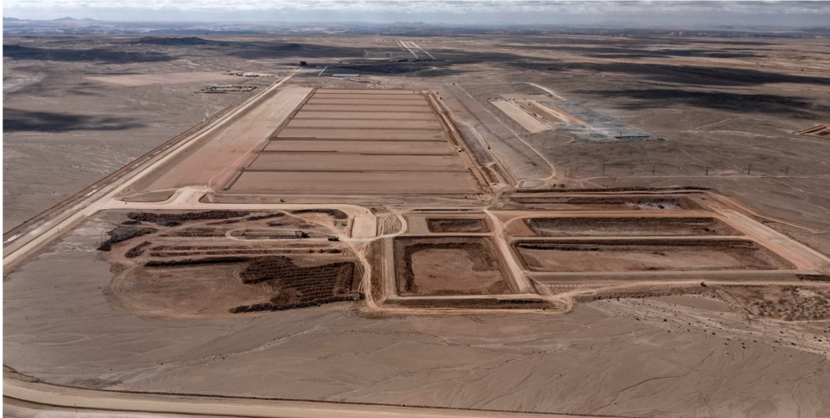
Figure 2: The Etango Project footprint is becoming increasingly visible as earthworks advanced across the heap leach pad, process solution ponds and wet plant terraces.
