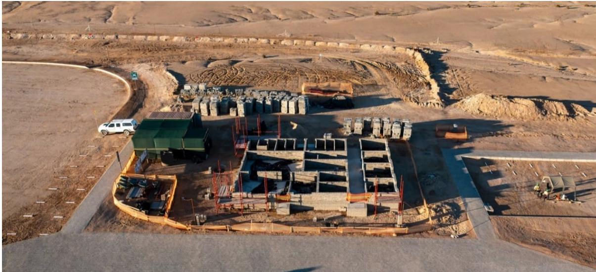
Figure 6: Aerial view of the Etango gate house being built by local Namibian-owned SME contractors.
