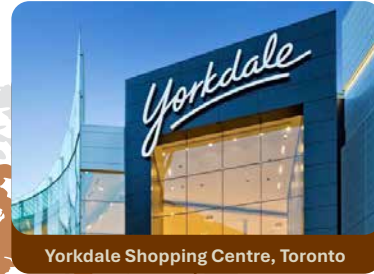
Yorkdale Shopping Centre, Toronto
