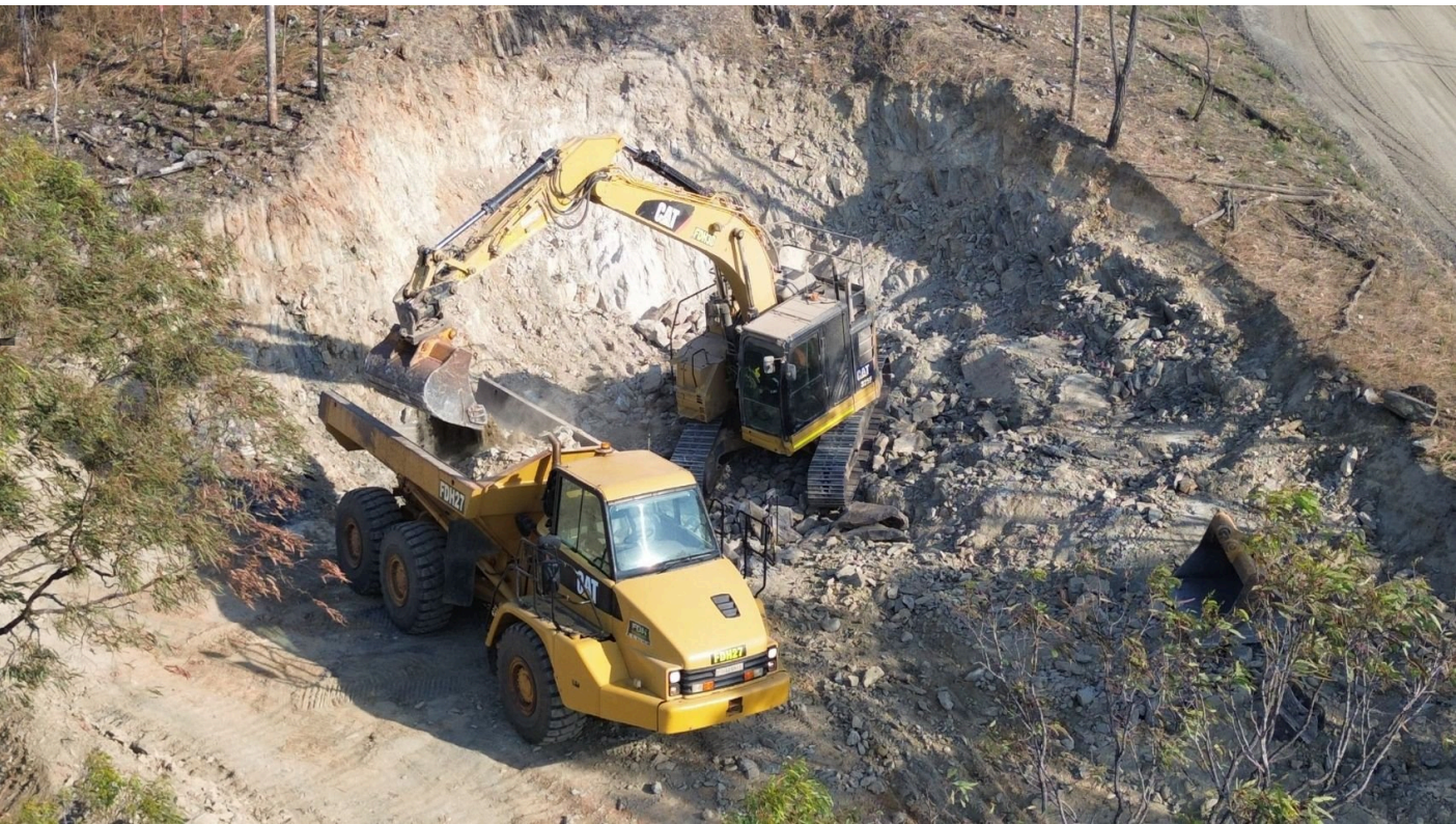
FIGURE 7 — BULK SAMPLING ACTIVITY UNDERWAY AT THE WATERSHED PROJECT
