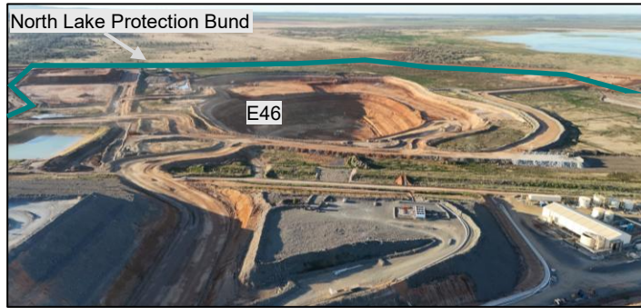
August 2026 - North Lake Protection Bund & E46
