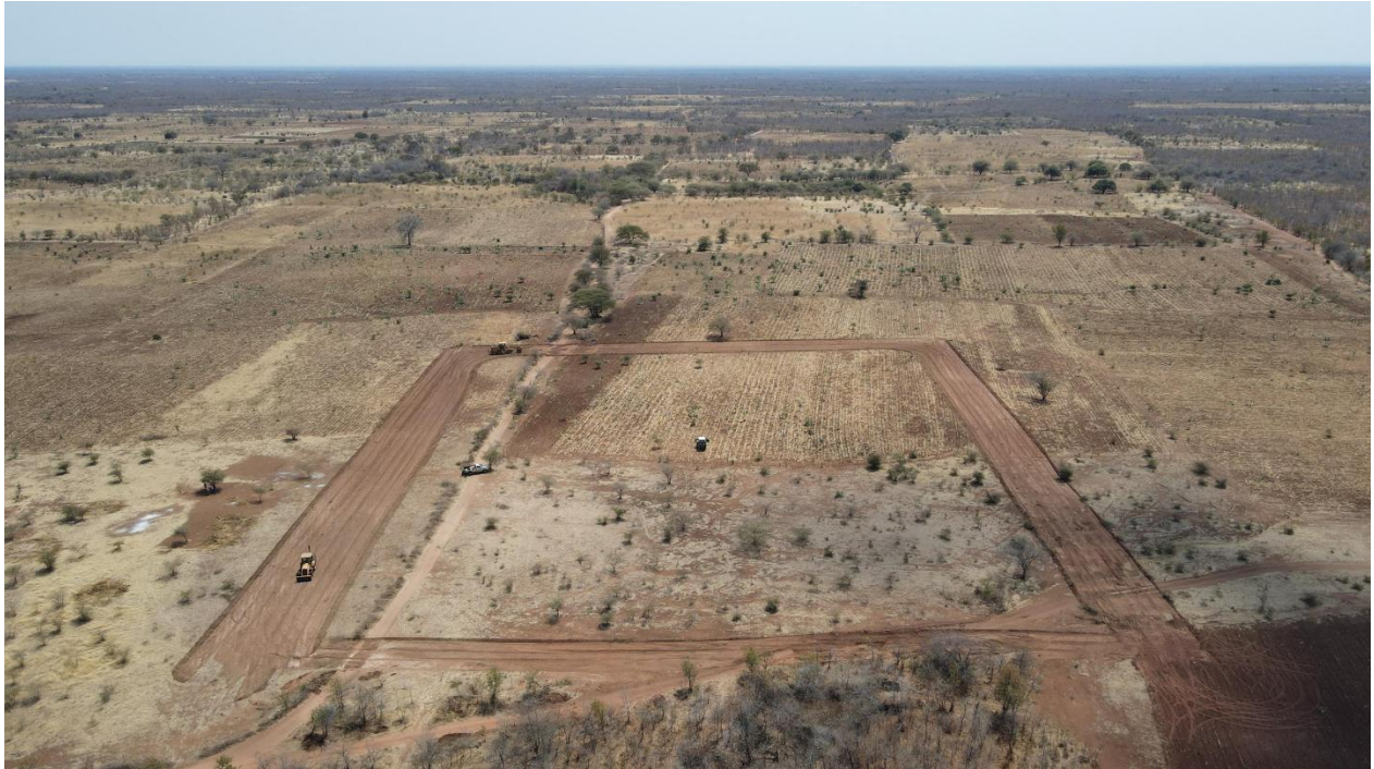
Figure 3 - Musuma-1 wellpad preparation
