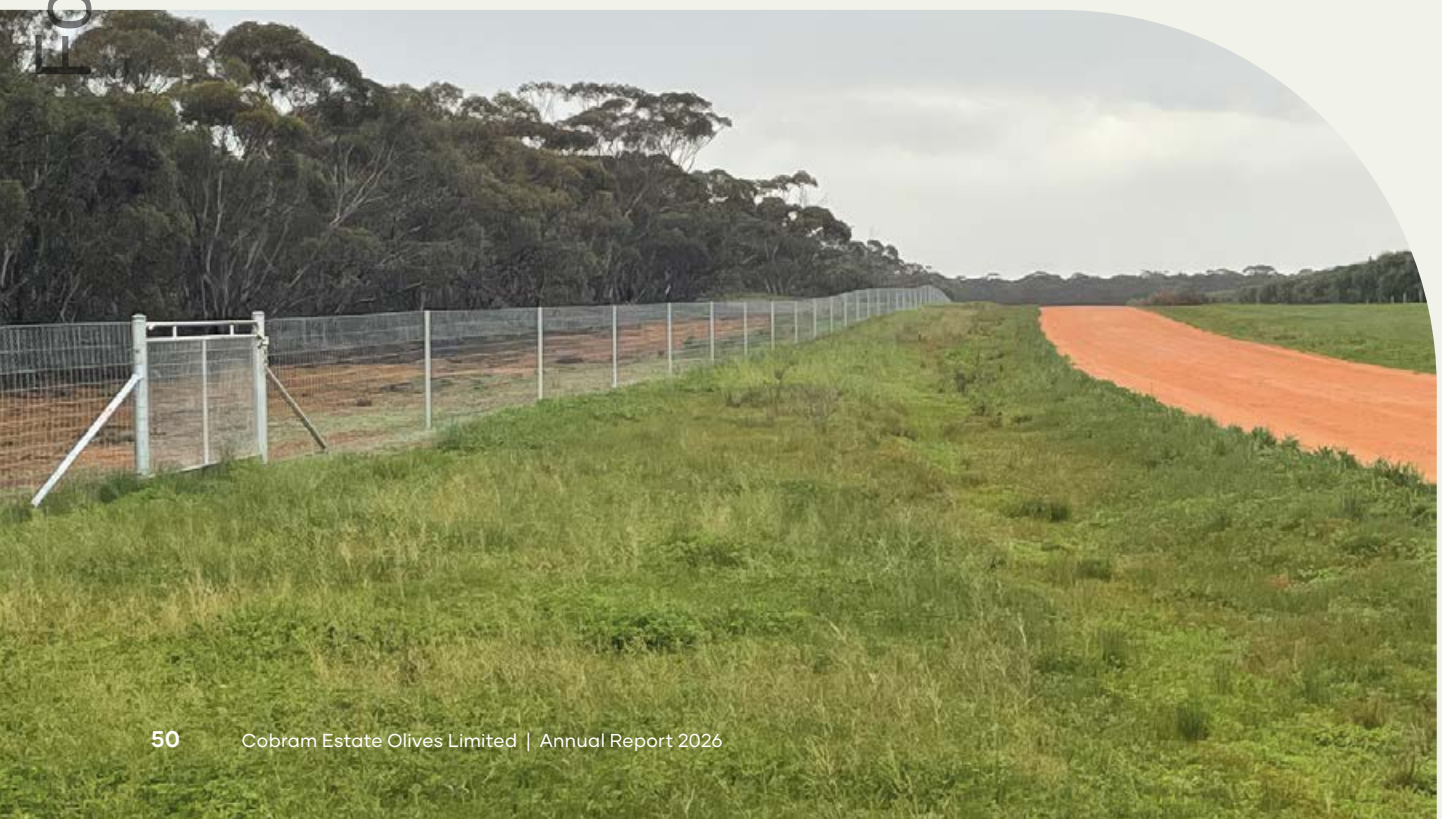
CONSERVATION EXCLUSION FENCE AT BOUNDARY BEND
