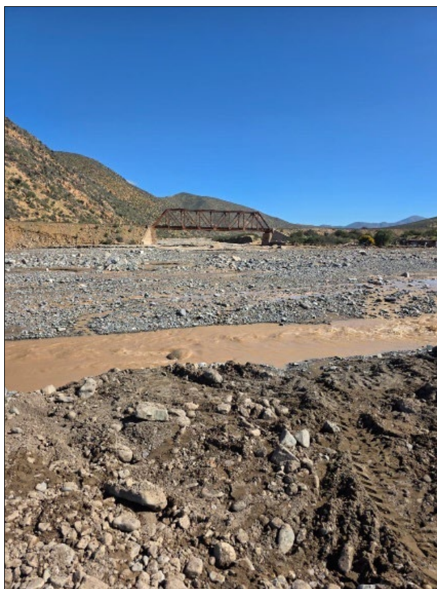
Figure 4. Los Loros Project main access route through Quebrada Santa Gracia, showing the affected section of the road following recent anomalous rainfall events.
