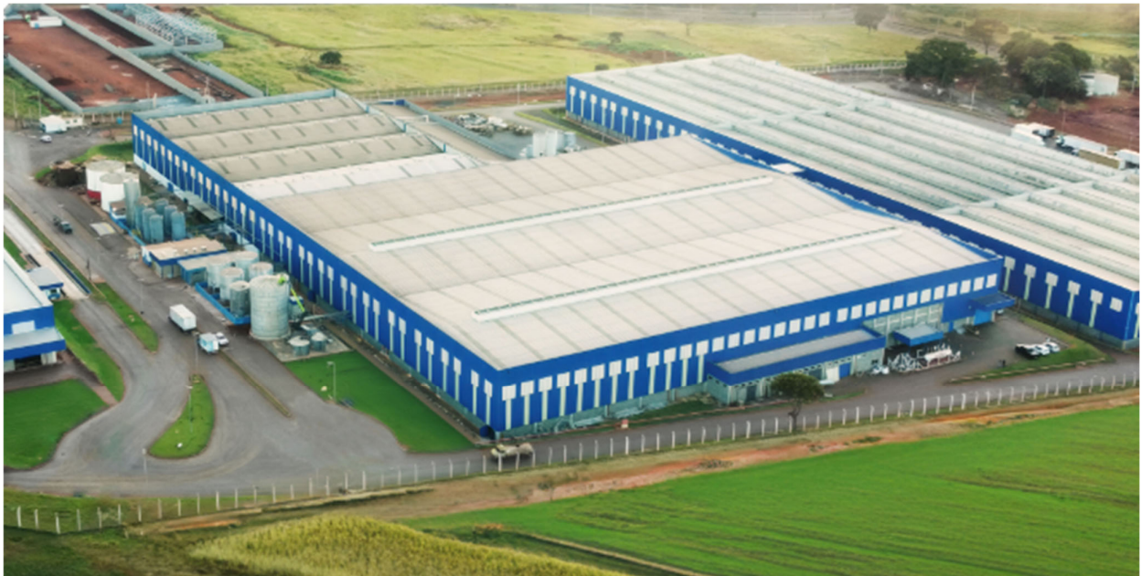
Figure 3 – photo of part of START's industrial complex at Uberlândia
