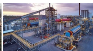
Kwinana Refinery Lithium hydroxide IGO 49%
