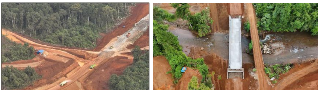
Sampala Mine construction activities
