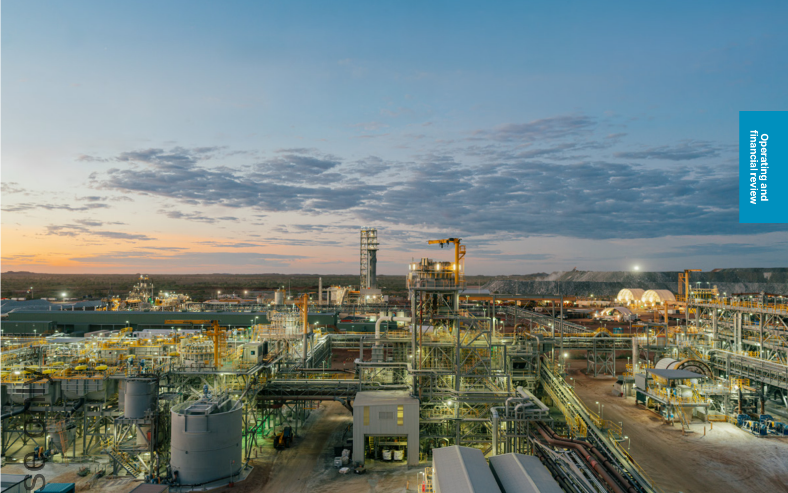
Aerial view of the Pilgan Plant and associated infrastructure at the Pilgangoora Operation
