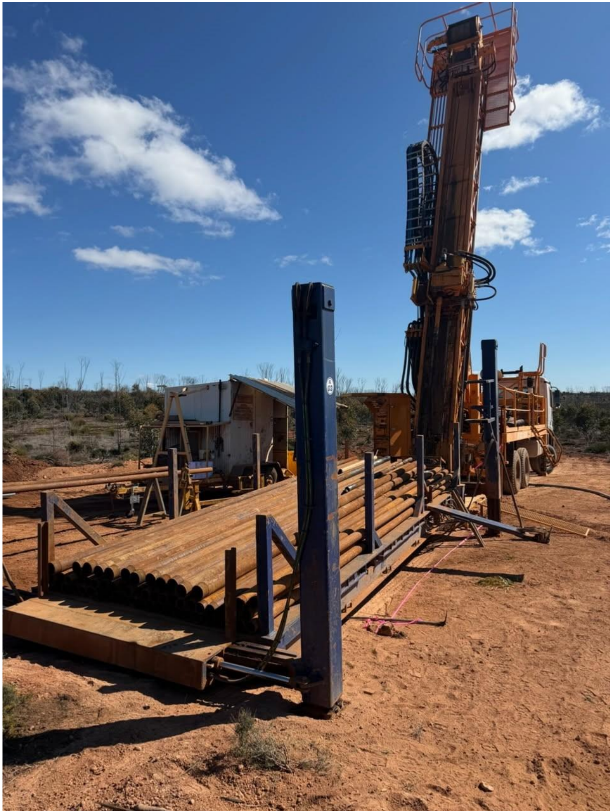
Figure 1 – Drilling Rig setup on first drillhole
