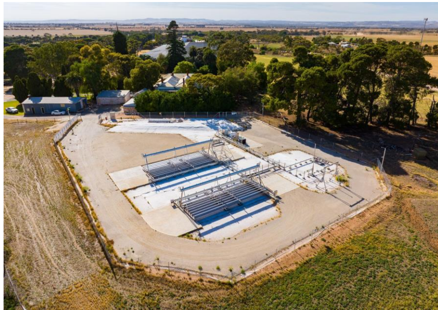
Sparc Hydrogen's SHARP Pilot Facility at Roseworthy, South Australia
