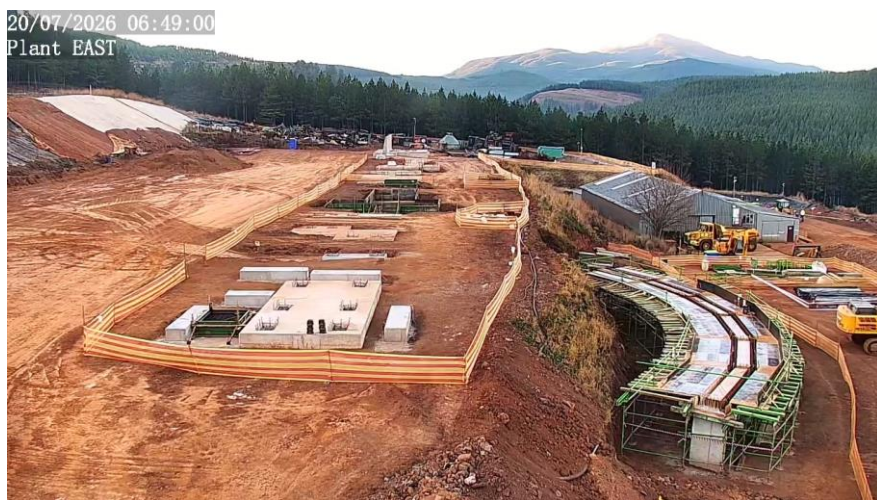
Figure 15: East view of the plant – indicating terrace walls and mill building
