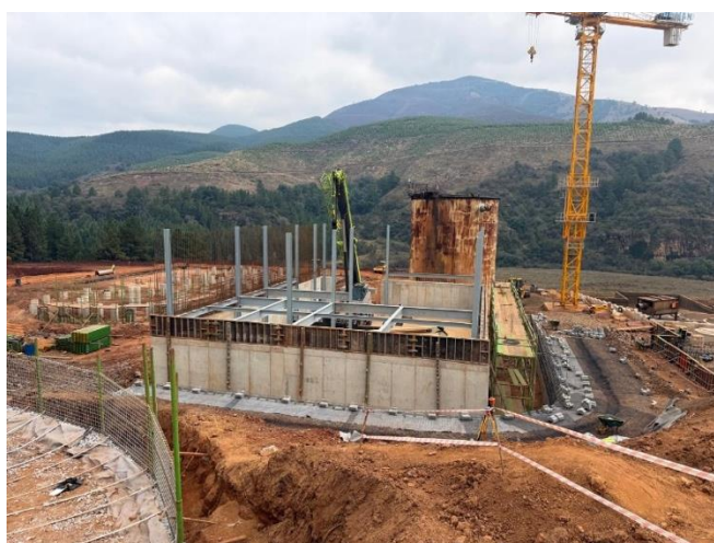
Figure 8: Gold Room construction continues - steel works
