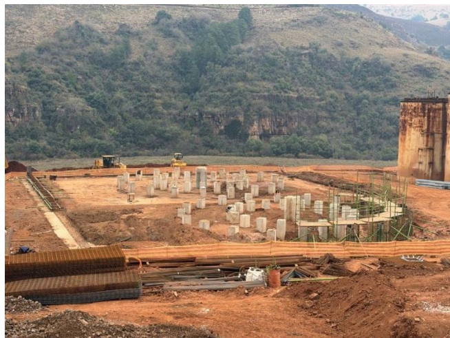
Figure 7: Thickener tank/processing area foundations
