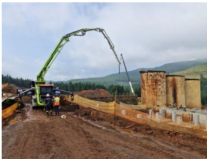
Figure 11: Concrete Pumping – Gold Room
