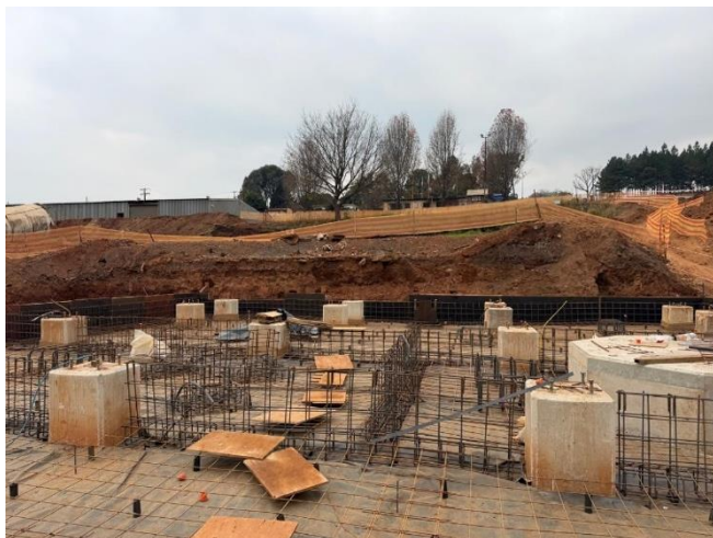
Figure 6: Elution circuit foundations
