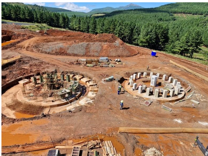
Figure 12: Thickener Tank foundations in progress
