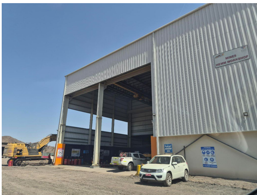
Figure 8 – Newly constructed Heavy Earth Moving Machinery (HEMM) Workshop
