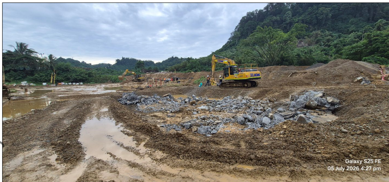
Figure 1: Pebble crushing circuit demolition
