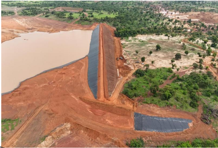
Figure 7: Water Storage Dam - Lined Spillway and Embankment
