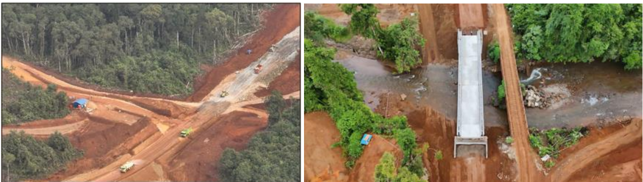
Sampala Mine construction activities
