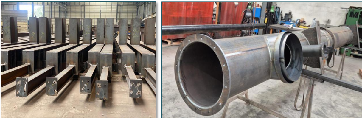
Fig .1. Steelwork underway - framework & piping for the dust extraction at Subantando Fertilizer Factory.
