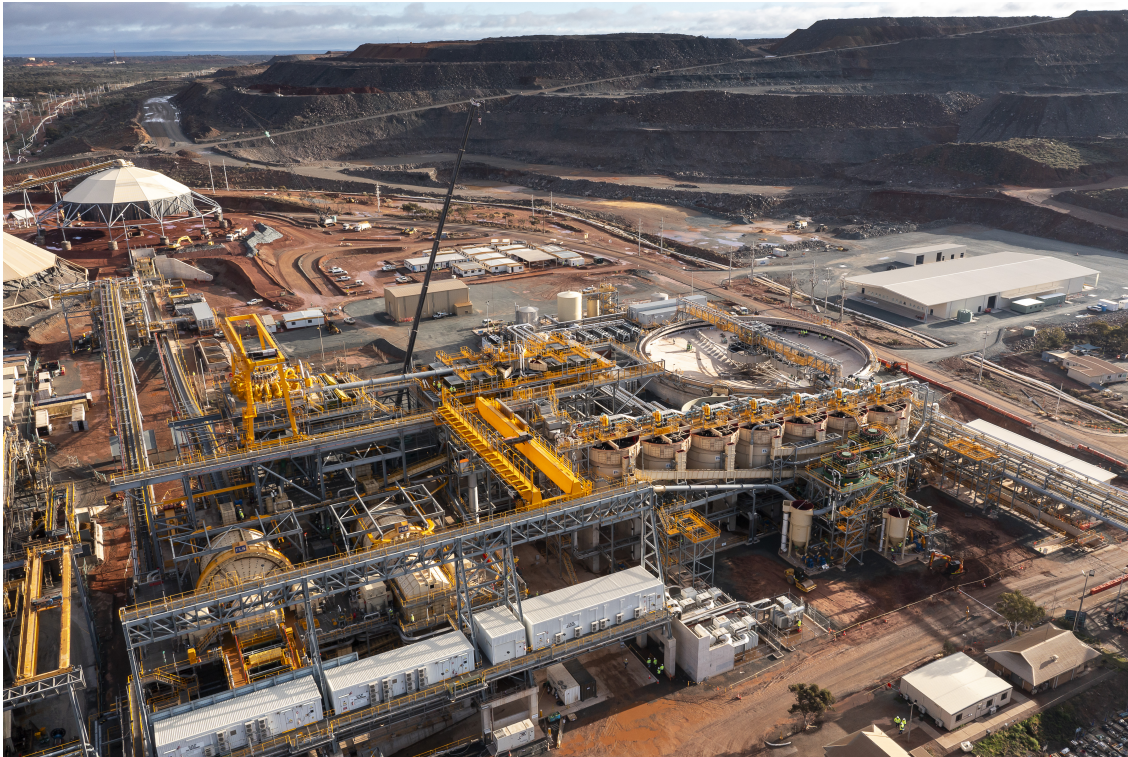
Figure 3: Aerial view of the Stage I expanded processing plant (foreground) and stockpiles (background).
