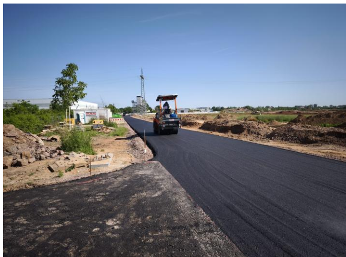
Figure 9: Road resurfacing post ICPP crossing work completion.
