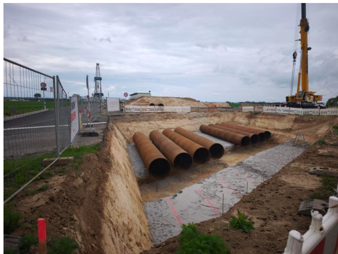
Figure 10: ICPP crossing to coincide with City of Insheim road refurbishment. See Schleiberg drill rig in the background.
