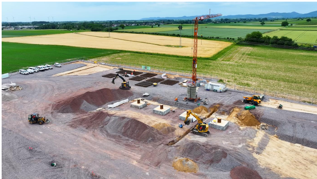
Figure 5: Construction works at the fourth well-site ahead of mobilisation of the second Vercana rig, known as V10, in H2 2026. Poured concrete for all four drilling cellars can be seen in the middle of the image.
