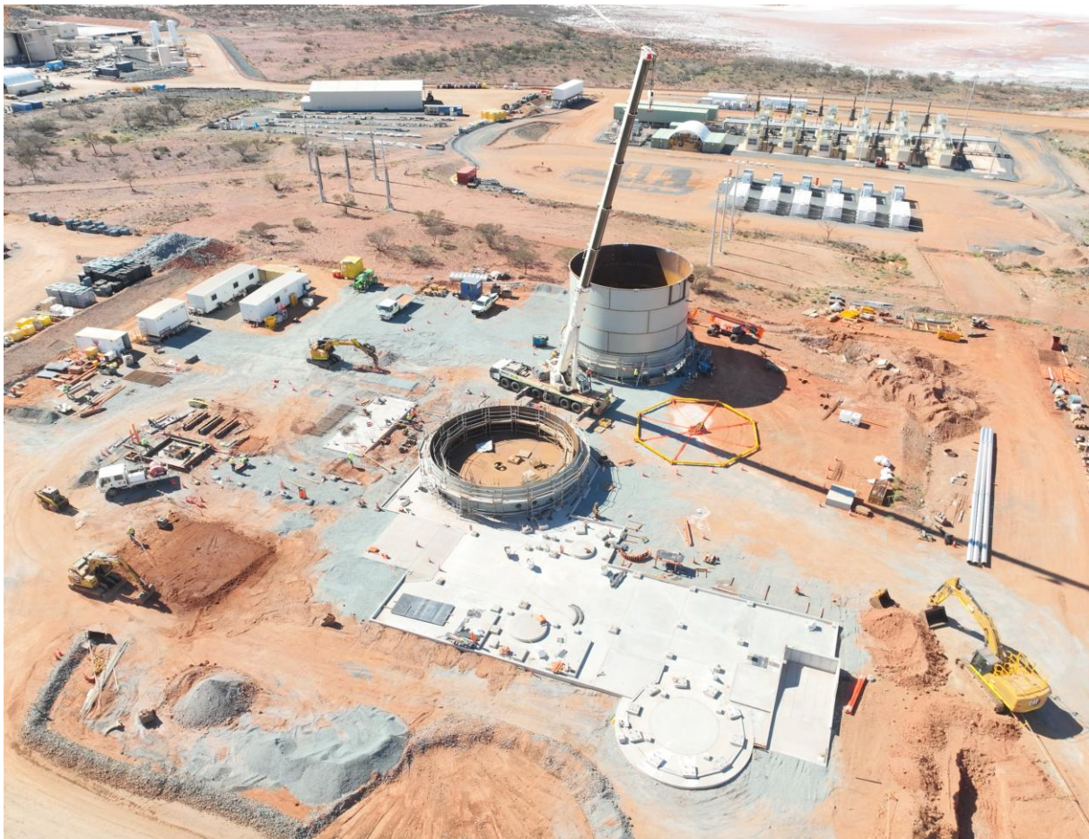
Figure 3: Paste Plant construction progress - 24 July 2026.
