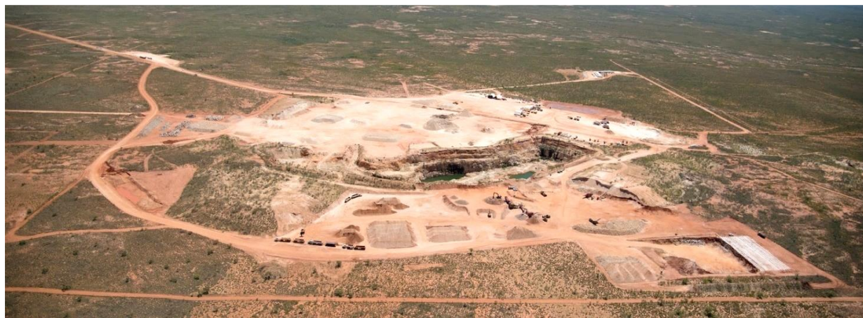
Figure 2:2 Pippingarra Quarry & Associated Infrastructure
