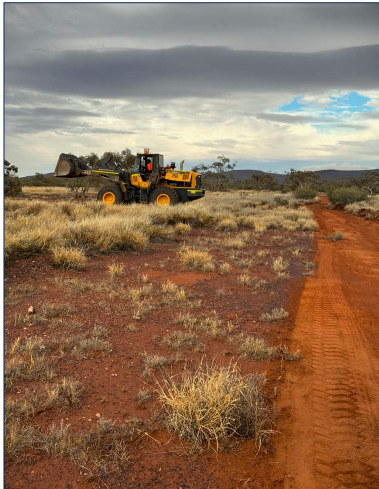
Figure 1. Ngaanyatjarra Civil completing clearing works for RC drilling at Nico's Wingellina Project.
