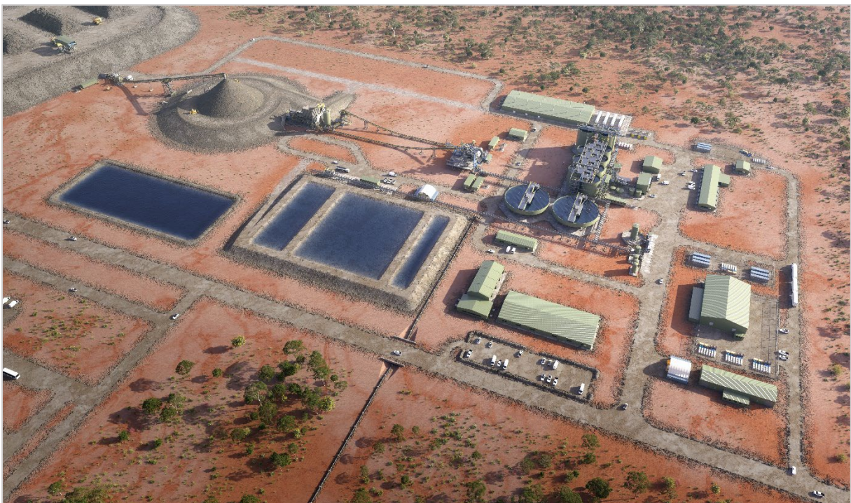
Figure 19: Overview of processing plant and supporting non-processing infrastructure
