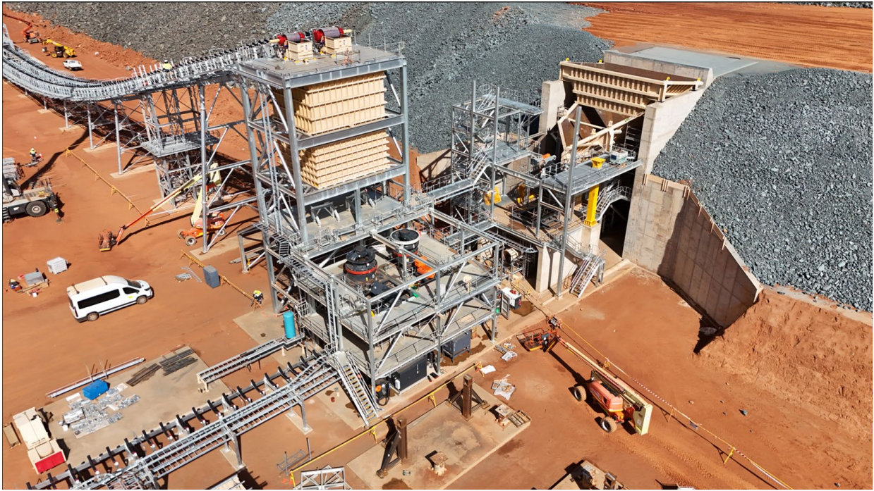
Primary/Secondary/Tertiary crusher building and ROM 2.
