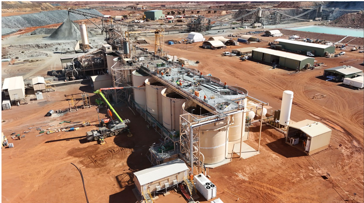
CIL circuit extension with top of tank steel sections in place.
