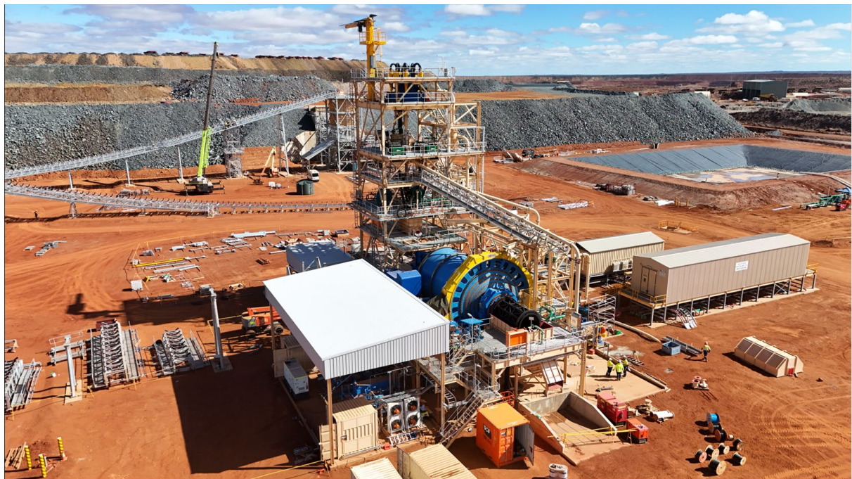
Mill area nearing completion.
