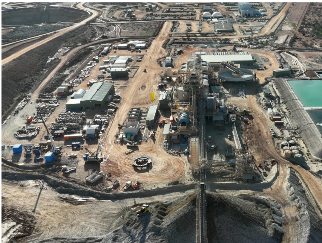
Figure 2: KoTH processing facility
