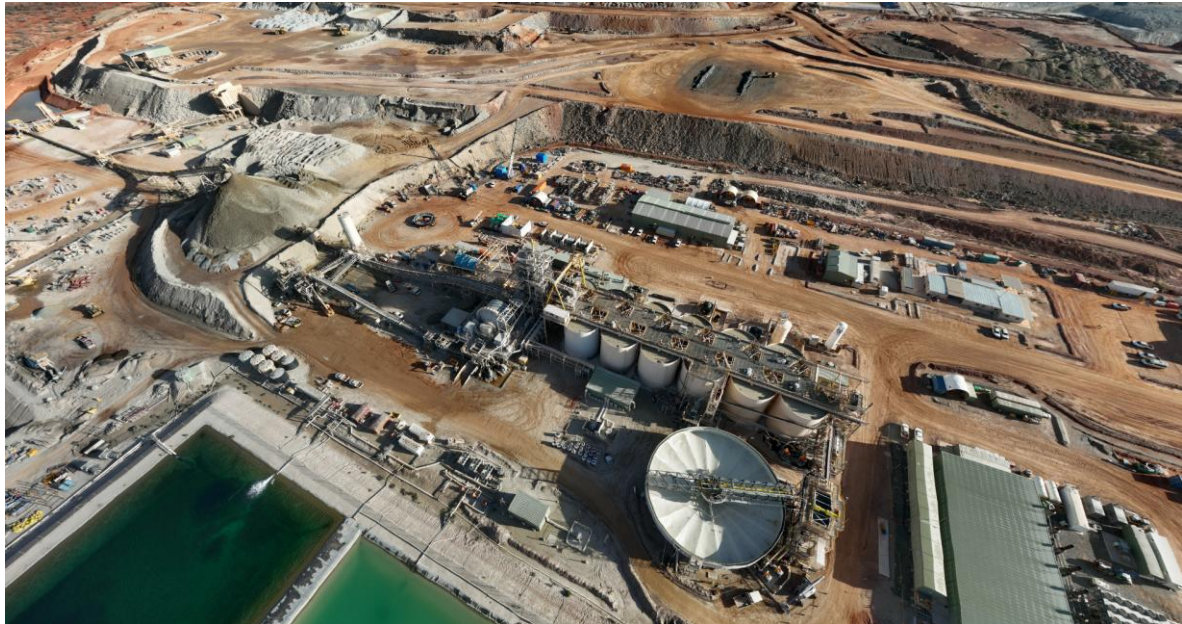
Figure 1: KoTH processing facility
