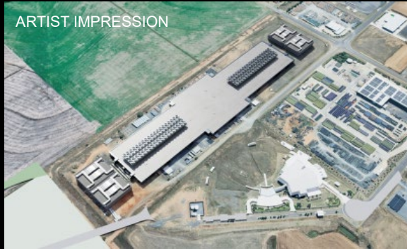
WELLCAMP TOOWOOMBA DC, EXPANSION
