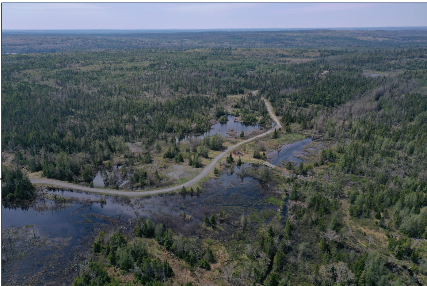
Figure 2: Existing historic 15-Mile project site
