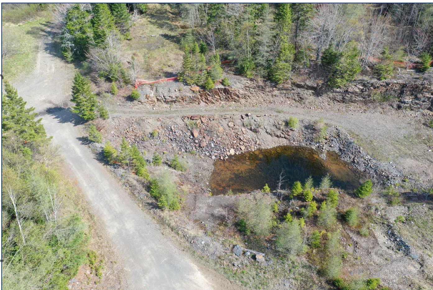
Figure 8: Existing historic Old Mitchell Mine site
