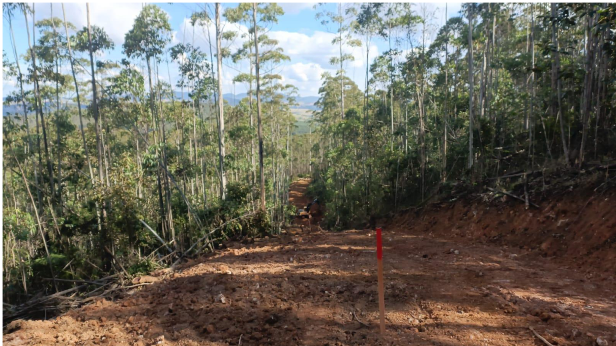
Figure 4: Drill pad site and access track at MDF Project. Note, there is no native vegetation in the project area; the vegetation is a eucalyptus plantation due for harvest in the near future.
