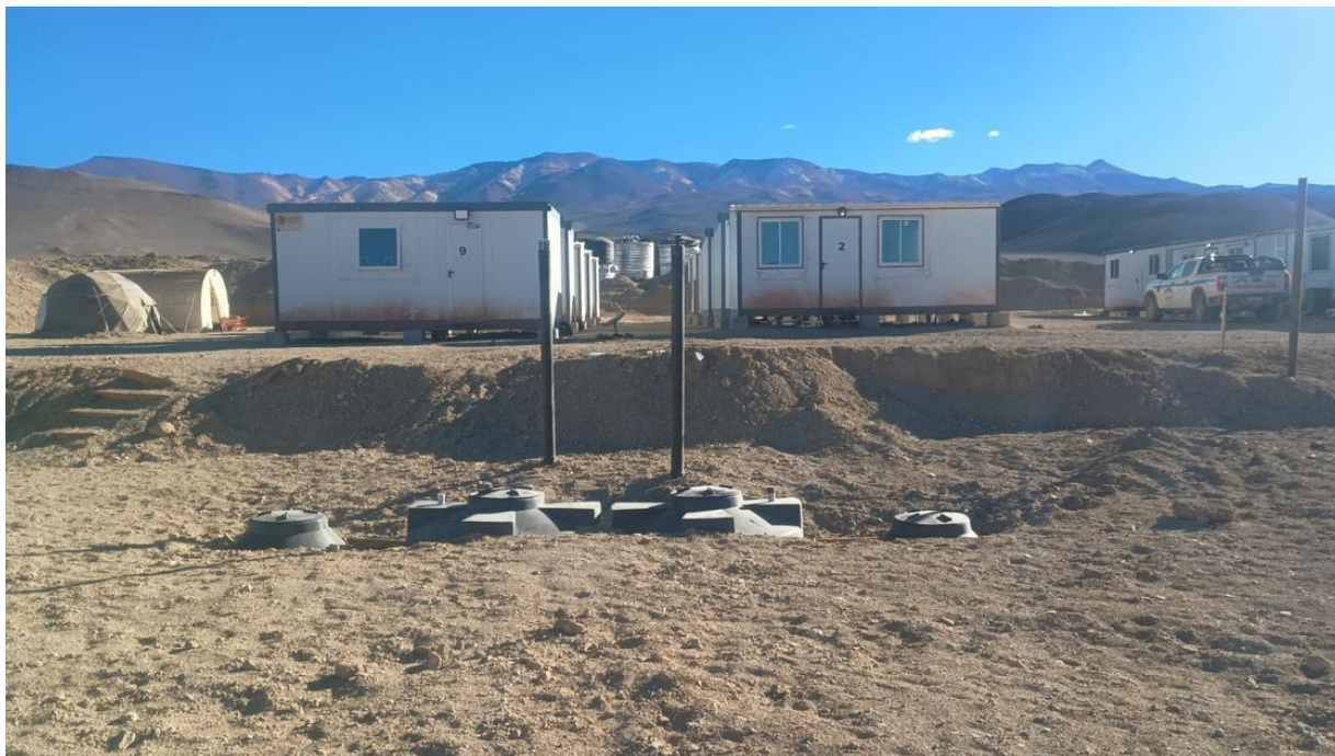
Figure 4 – Drilling Camp Established at Rio Grande Sur Ahead of Commencement of DDH-3.
