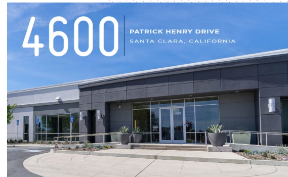
State -of-the -art facility in Santa Clara, California
