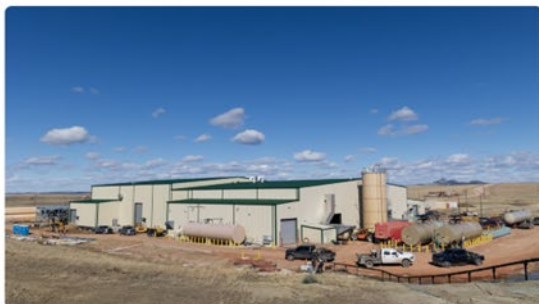
Central Processing Plant (Phase I & II)
