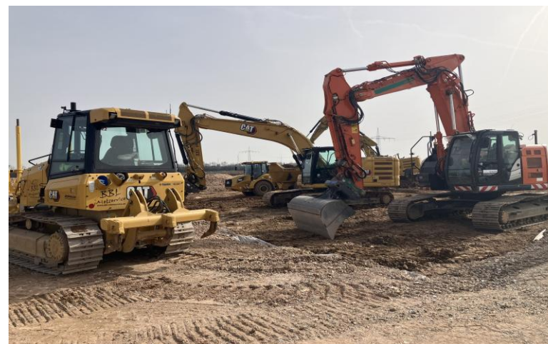
Construction at the integrated geothermal and lithium extraction site near Landau
