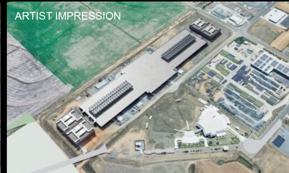
WELLCAMP TOOWOOMBA DC, EXPANSION
