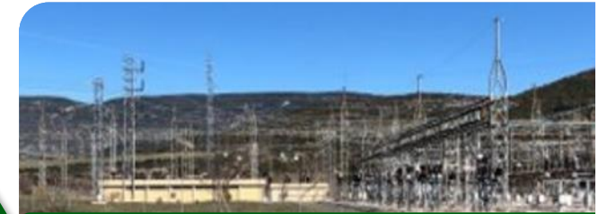
National Electricity Grid Substation in Sangüesa
