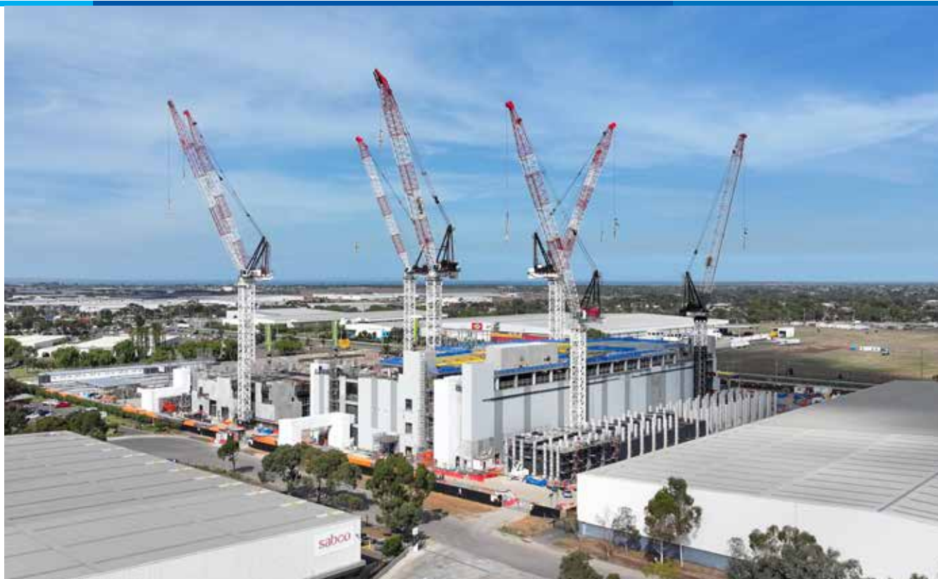
Construction at CDC's Laverton campus, Melbourne.
