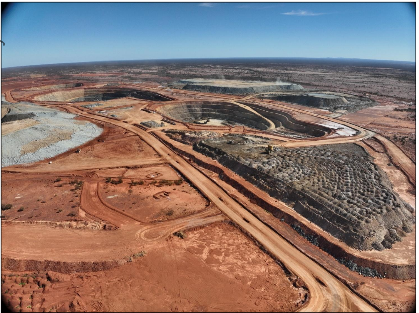
Figure 5: Cue open pit mining - Break of Day (left) and Lena (centre)
